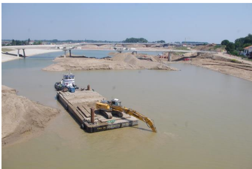
Figure 8: Room for the river Waal - Reconstruction of a new river arm, protecting the city of Nijmegen, The Netherlands (Source: Mathias Scholz, UFZ)
